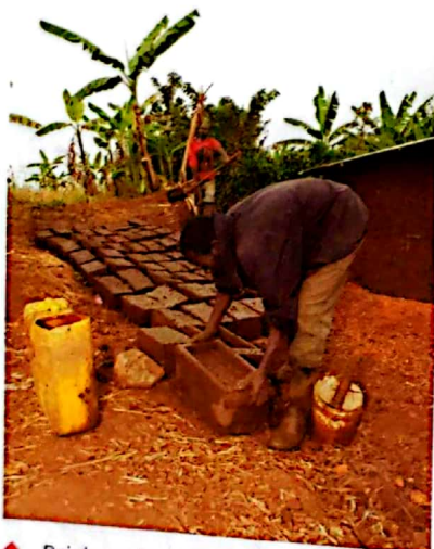
↑ Brick making in Rwanda.
